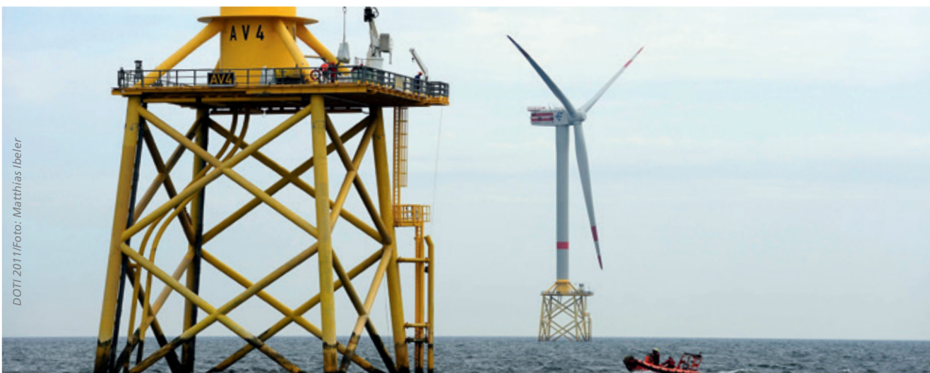
Jacket foundation of the „alpha-ventus“ wind farm
